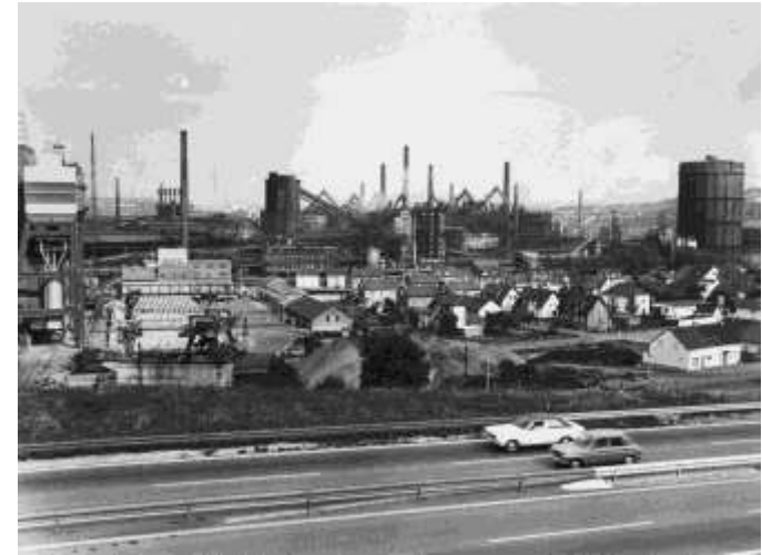
Stahlwerk Röchling, Foto: LA Saarland, B 1781/74 D © NL Erich Isenhuth, STA St. Ingbert.
